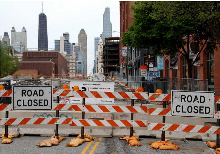
A road closure due to ongoing construction of the Chicago Avenue bridge on April 28. ANTONIO PEREZ/CHICAGO TRIBUNE
