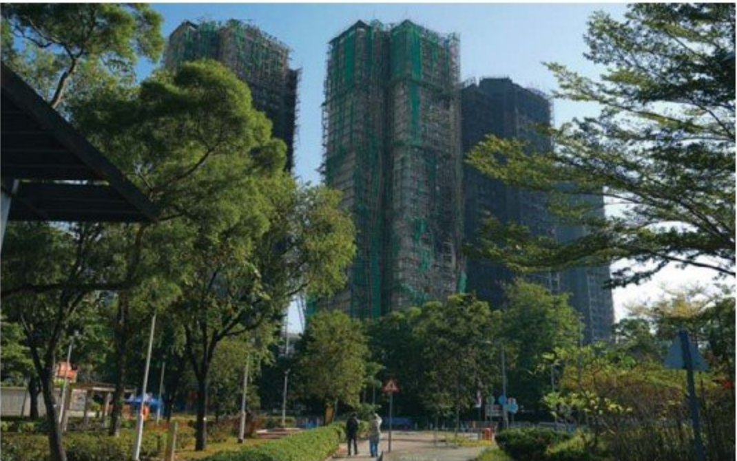
Wang Fuk Court in Tai Po nearly three weeks after the fire. Photo: Sam Tsang
