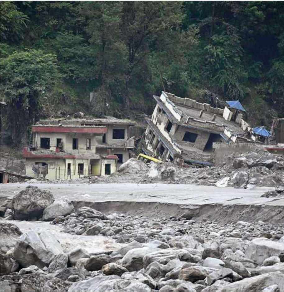
Trail of destruction: Damaged houses covered in sludge in the aftermath of the flash flood in Nepal’s Rasuwa district. AFP
