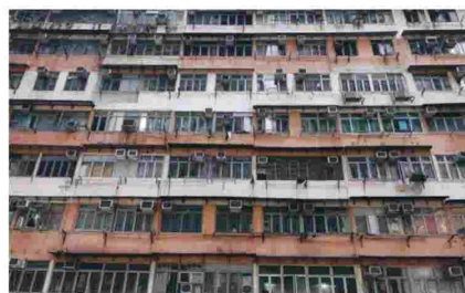
An old residential building in San Po Kong, typical for Hong Kong. Photo: Edmond So
