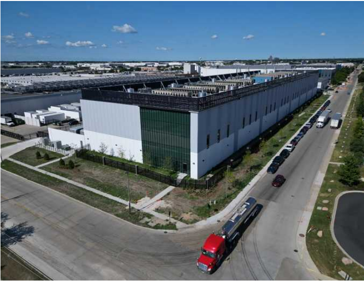
The EdgeConneX CHI03 data center on July 22 in Elk Grove Village. . STACEY WESCOTT/CHICAGO TRIBUNE
