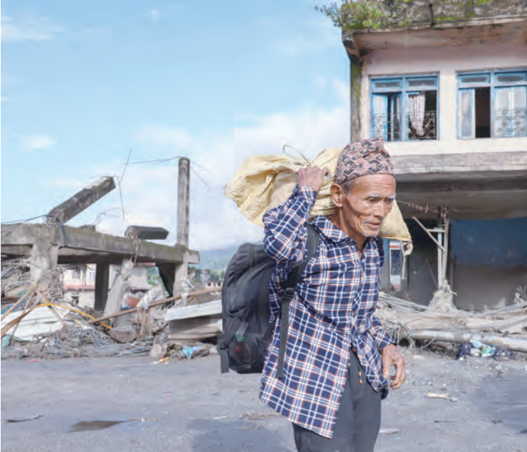
A man carries personal belongings on his back as he walks past flood-damaged houses, following deadly flash floods and a mudslide, in Devighat, Nuwakot district, Nepal. — Reuters
