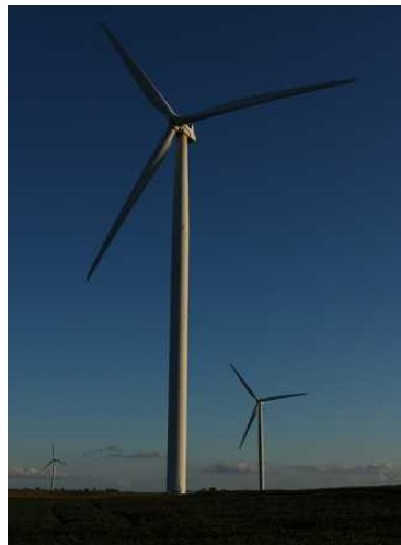
Wind turbines generating renewable energy rise above farmland Aug. 20, 2025, in Gibson City. JOHN J. KIM/TRIBUNE
