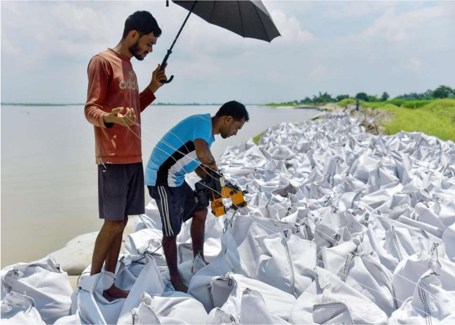
Workers prepare geo bags to prevent erosion of the Brahmaputra river bank at Borakhat village, in Kamrup district of Assam on August 7. ANI
