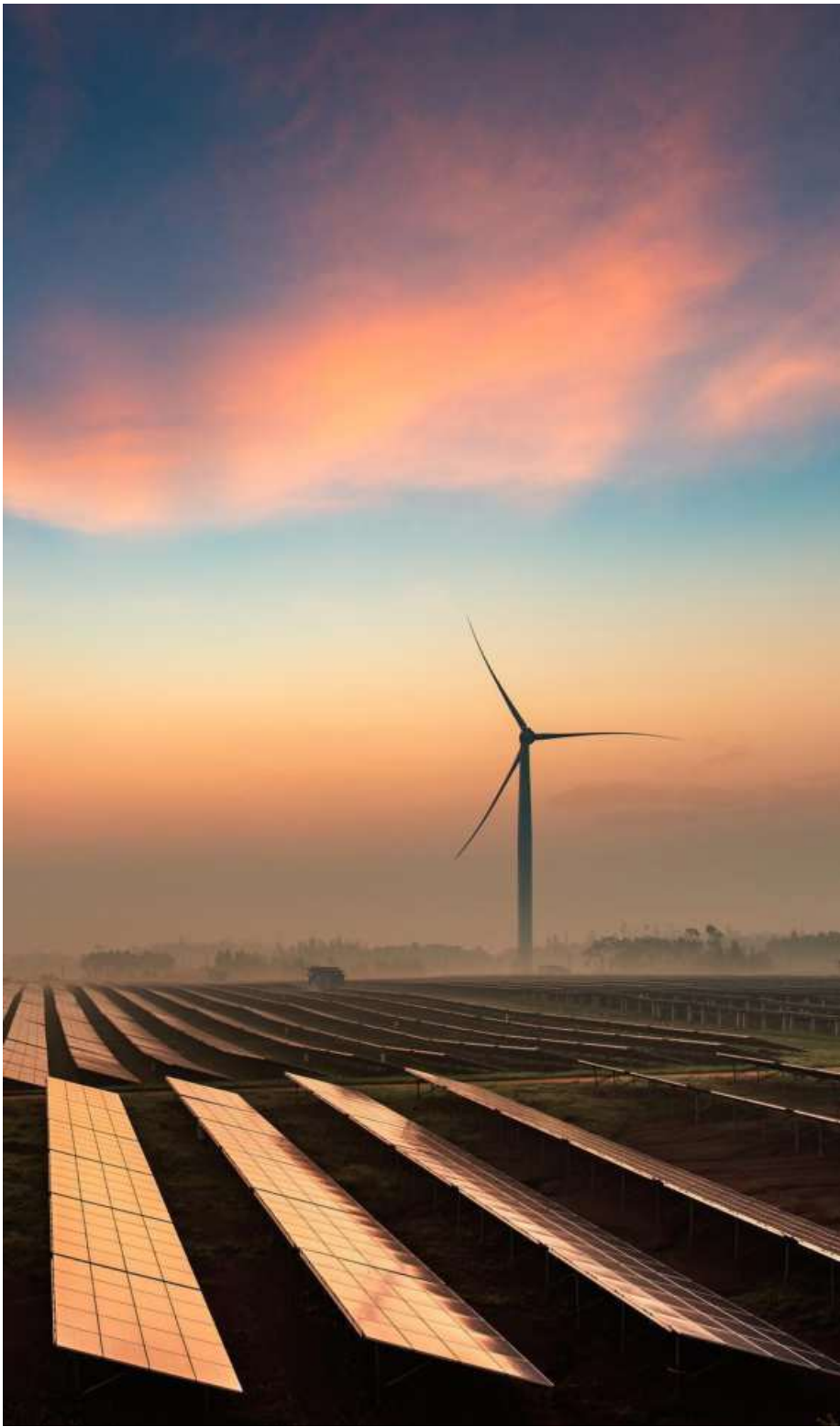
Powering up: A successful electrification programme hinges on affordable and reliable renewable electricity supply. GETTY IMAGES
